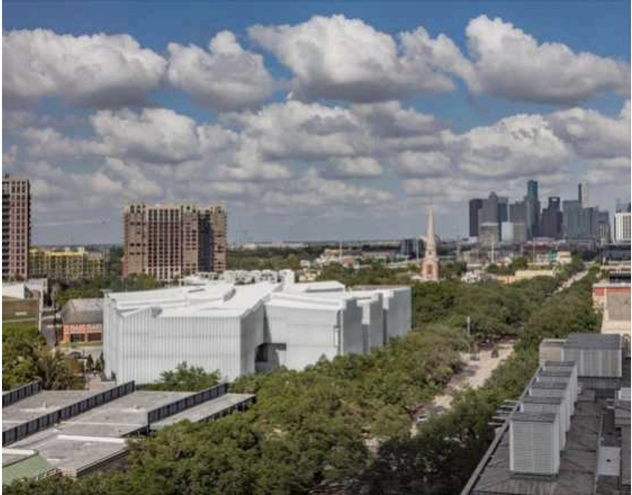
The Houston Museum of Art, designed by Stephen Holl, 'Architect of Light'. Expect to become Houston's premier landmark. Photographed by Richard Barnes. [Picture MFAH]
