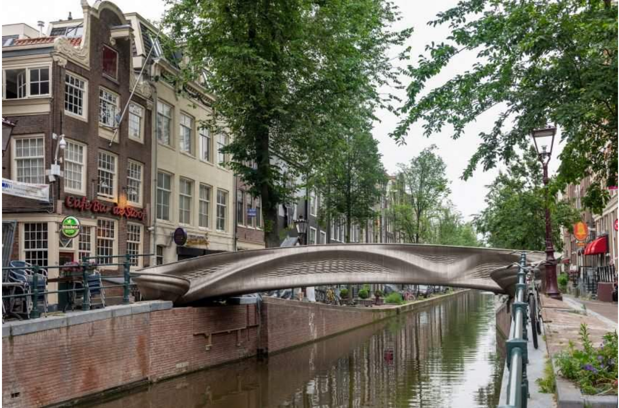
Top: MX3D Bridge is located in the Red Light District. Above: it was 3D-printed from stainless steel
