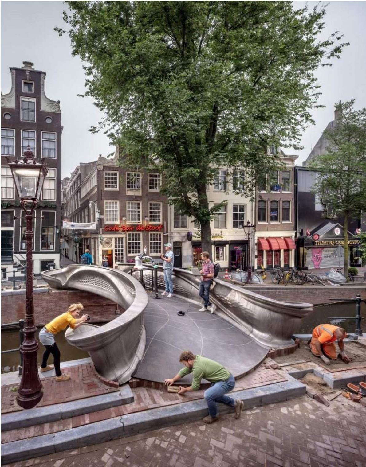
It was made from 4,500 kilograms of stainless steel. Photo is by Thijs Wolzak
