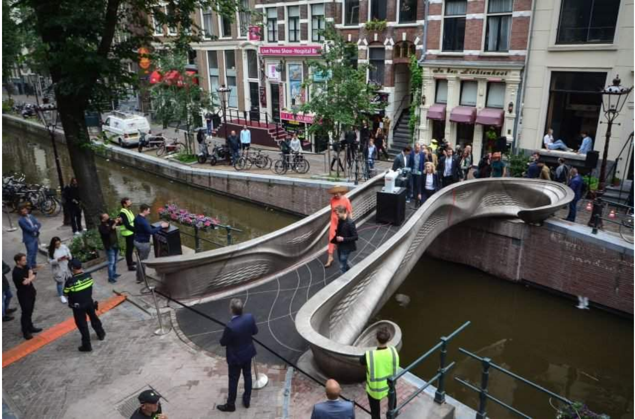
The bridge was constructed using robotic printers. Photo is by Adriaan de Groot
